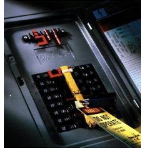
Locked out circuit breaker
